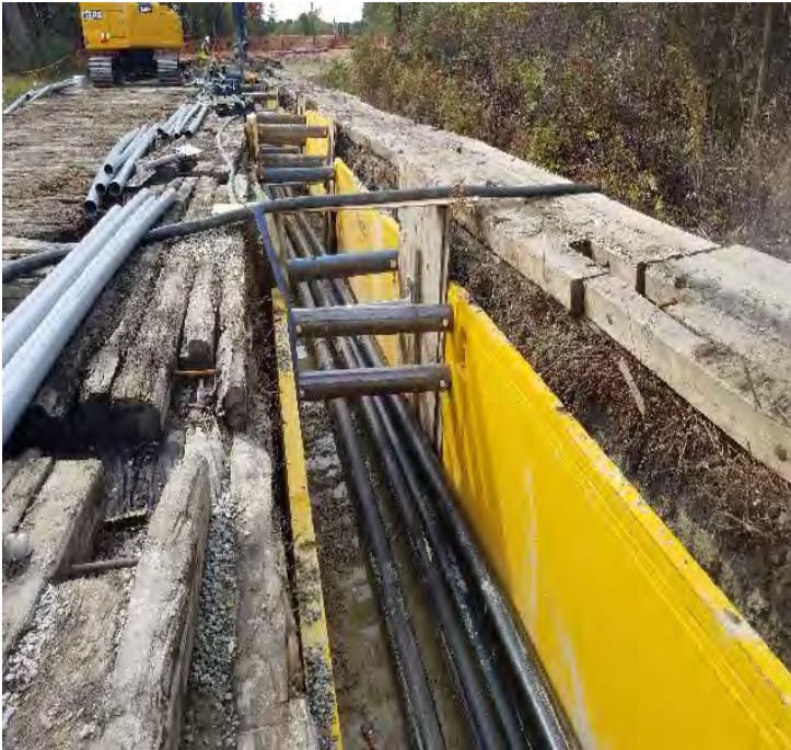
Fig 19: Installing pipe in trench at Str. 106. Viewing west. (10-8-19).
