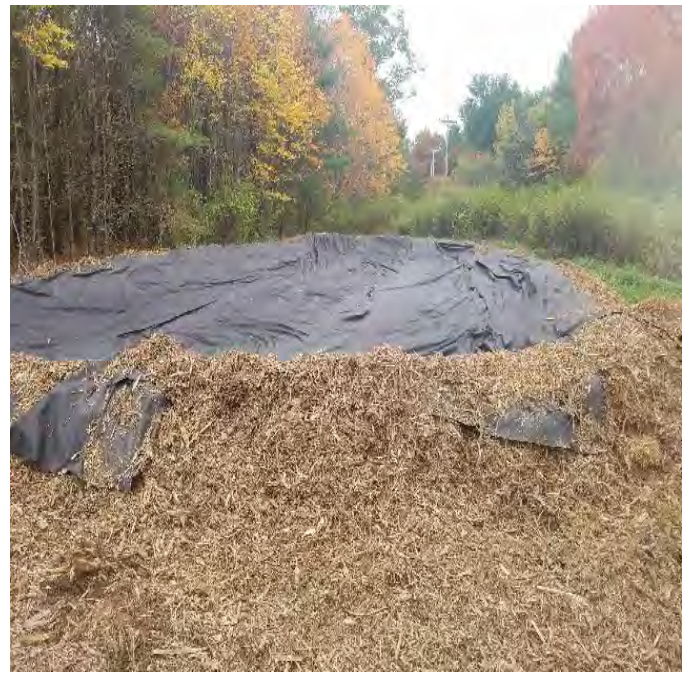
Fig 22: Dewatering basin at Str. 48. Viewing southwest. (10-9-19).
