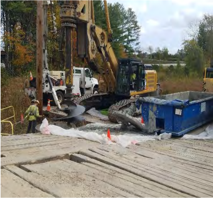
Fig 13: MJ drilling Str. 117. Viewing east. (10-7-19).
