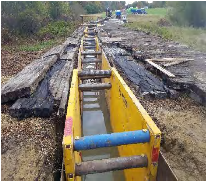
Fig 1: Trenching from Str. 106. Groundwater accumulation in trench. Viewing east. (10-03-19).
