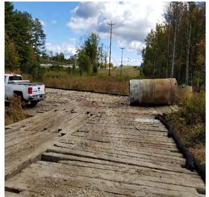
Fig 8: Timber matting at Str. 117, prepping to drill. Viewing east. (10-04-19).
