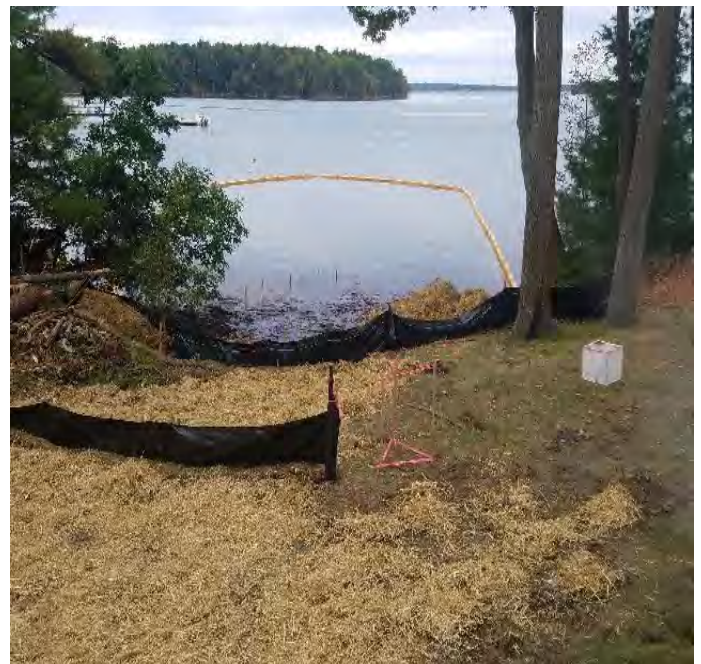
Fig 4: Sediment controls installed at the Beswick property in Newington. Viewing west. (10-03-19).
