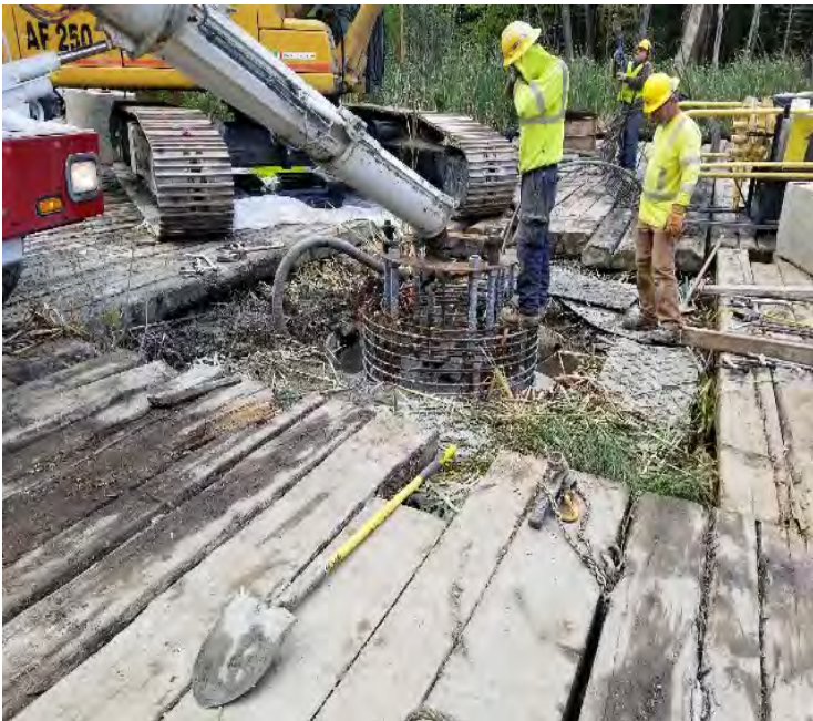
Fig 7: Final concrete pour for Str. 116 foundation. Viewing southwest. (10-04-19).
