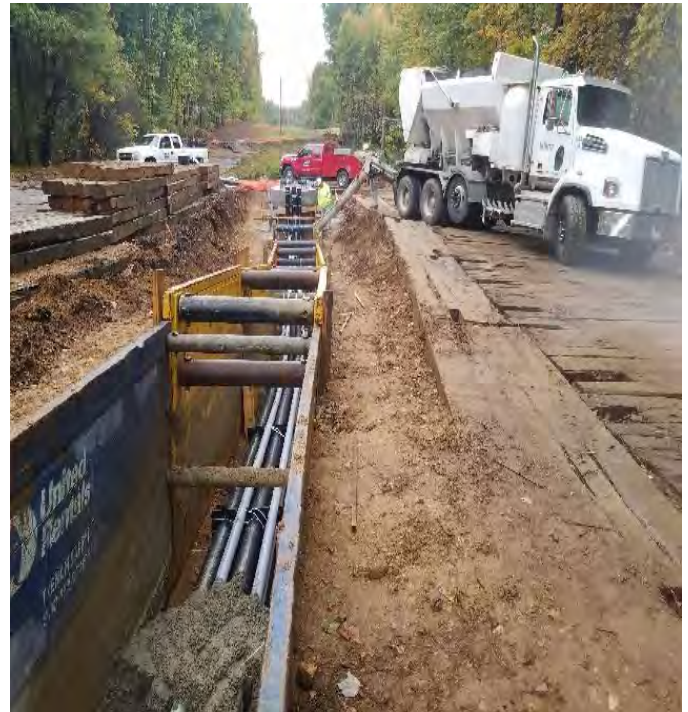
Fig 16: Duct bank in trench at Str. 107. Viewing east. (10-8-19).
