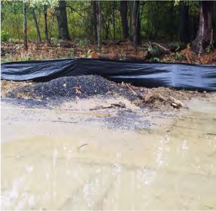
Fig 17: Cold patch asphalt at Flynn pit. Needs to be removed. Viewing south. (10-8-19).
