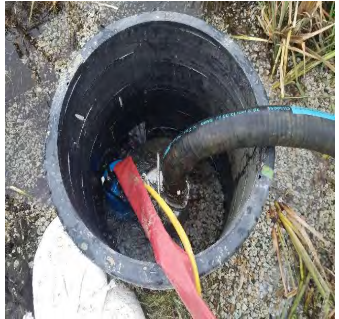
Fig 10: Stream bypass pump, upstream in Knights Brook. Viewing south. (10-7-19).
