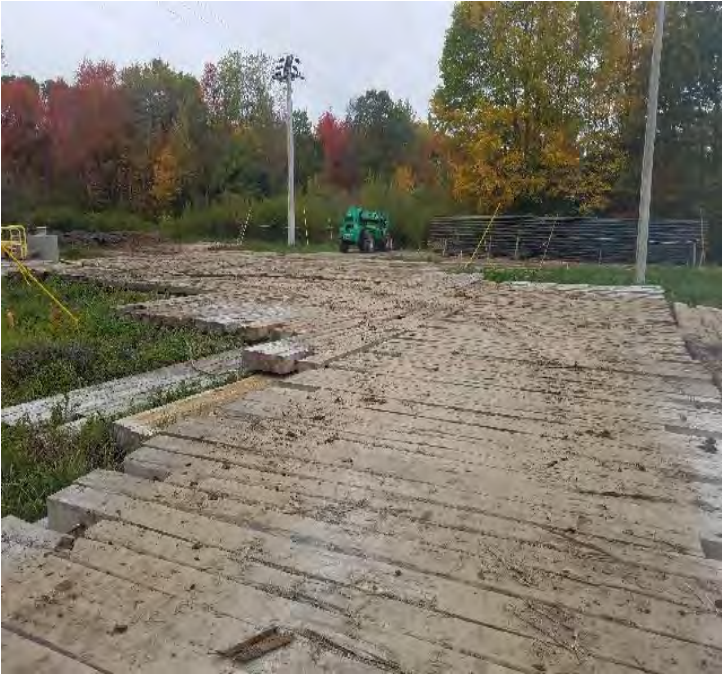
Fig 21: Work pad at Str. 48. Viewing west (10-9-19).
