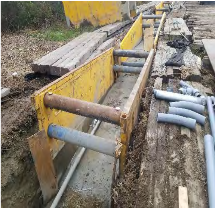
Fig 25: Duct bank in trench at Str. 106. Viewing east. (10-9-19).
