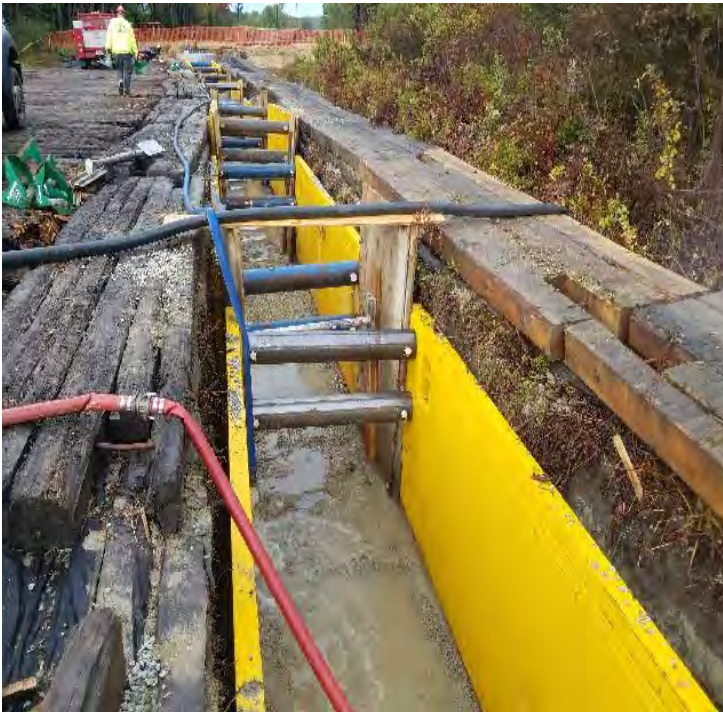
Fig 15: Dewatering trench at Str. 106. Viewing west. (10-8-19).
