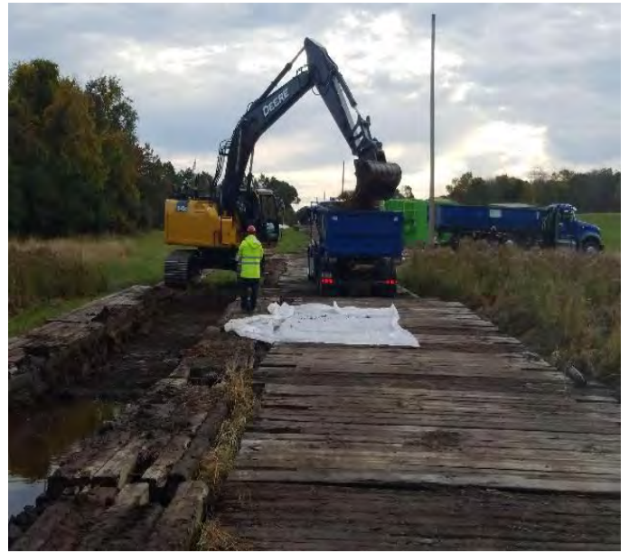
Fig 2: Stripping topsoil in wetland NW16. Viewing east. (10-03-19).
