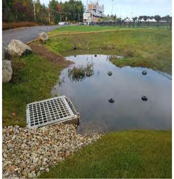
Fig 18: Rain garden at UNH. Viewing east. (10-8-19).
