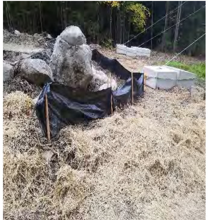
Fig 24: Silt fence repaired at Str. 29. Viewing east. (10-9-19).
