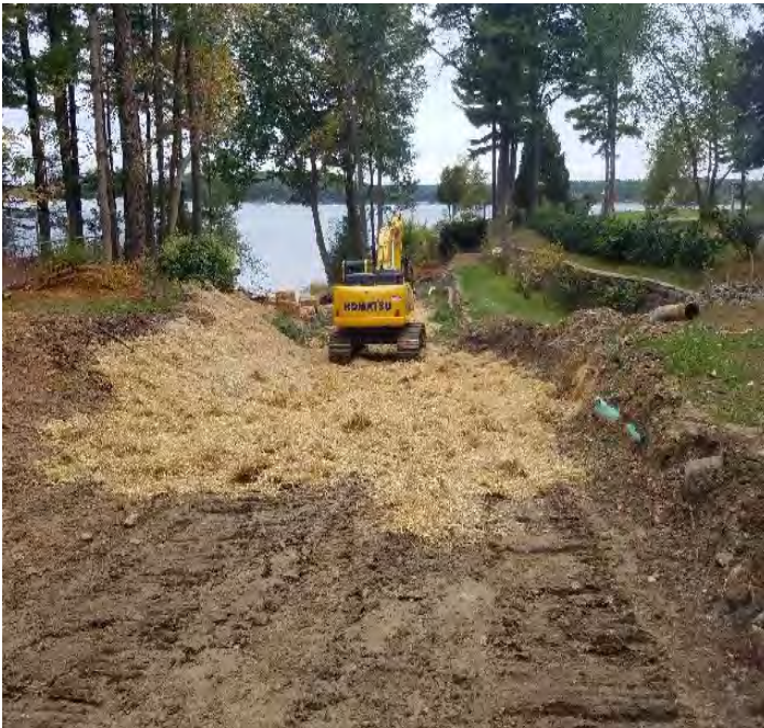
Fig 3: Exposed soils mulched at the Beswick property in Newington. Viewing west. (10-03-19).
