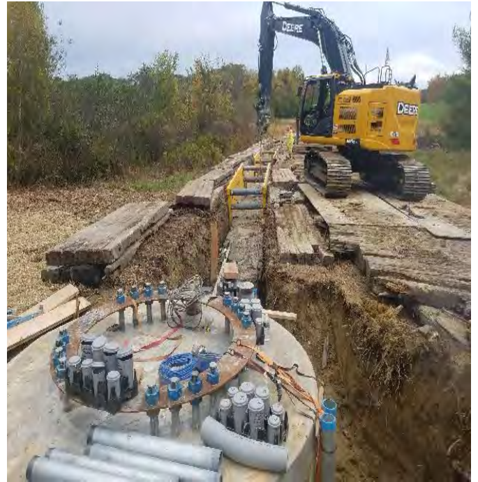
Fig 26: Removing trench boxes at Str. 106. Viewing east. (10-9-19).
